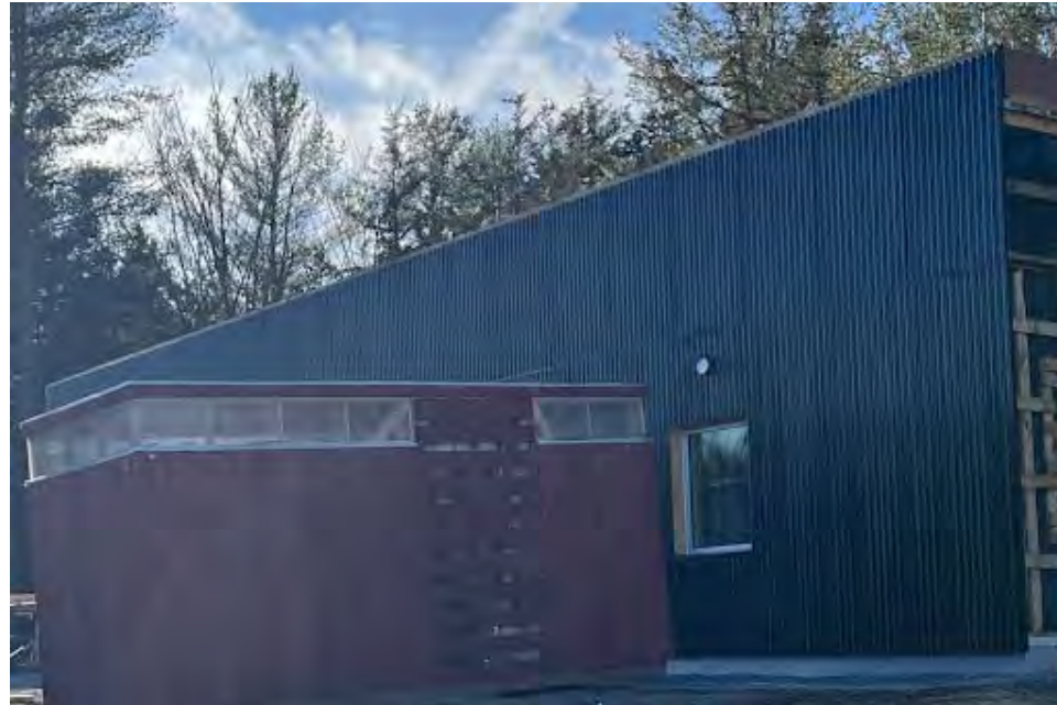
North Elevation with Shed
